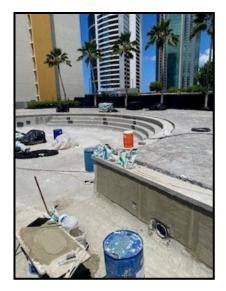
In June, July and August all spalling was repaired and patched, and a new concrete coping beam installed around the deck side of the pool.
