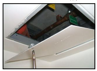
valves isolate the water supply to all the bathroom fixtures. They do NOT isolate the kitchen, the refrigerator ice maker, or the washer/dryer water supply.
