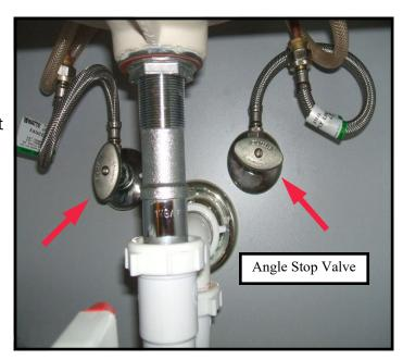
These valves need to be exercised. The plastic pipe is behind the valve inside the wall. If the valve handle does not turn easily, the plastic can break.
